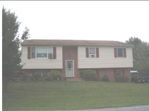
split level – 2 full floors of living area with entrance at grade between the lower level floor below grade and upper level floor 4 feet above grade
