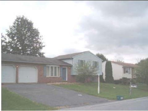
bi – level - similar to split level with entrance at grade level, lower level floor on one side, a grade level floor, and an upper level floor above grade level
